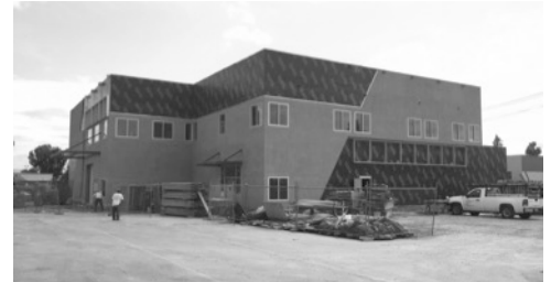
District builds a new Central Kitchen for cost-effective and fresh student meals.
